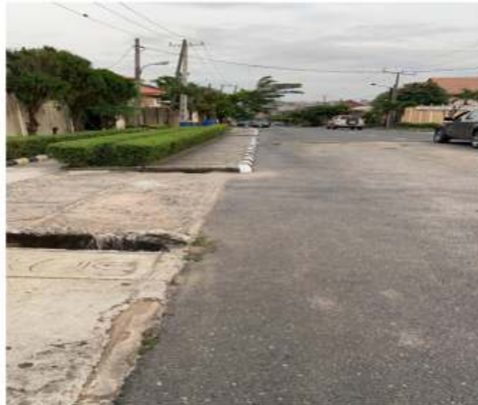
Good practice of walk way and drive in ramp
